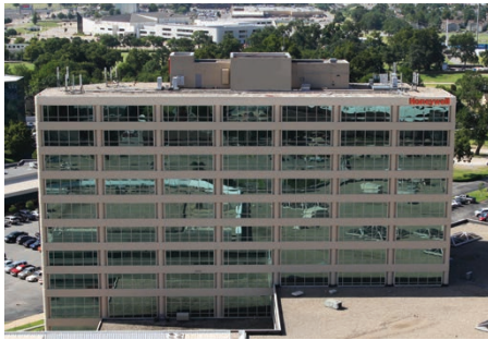
Honeywell UOP Callidus headquarters - Tulsa, Oklahoma. USA
