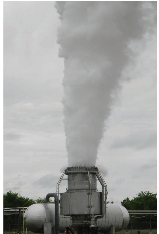
Internal Steam Flare Tip High Steam Flow Testing
